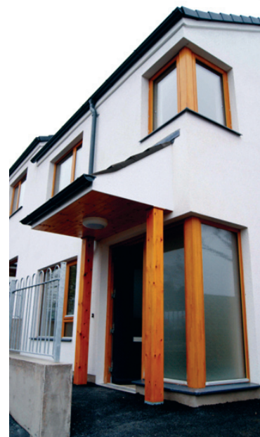
Social Housing Project using Hempcrete & Timber, Antrim N.Ireland
